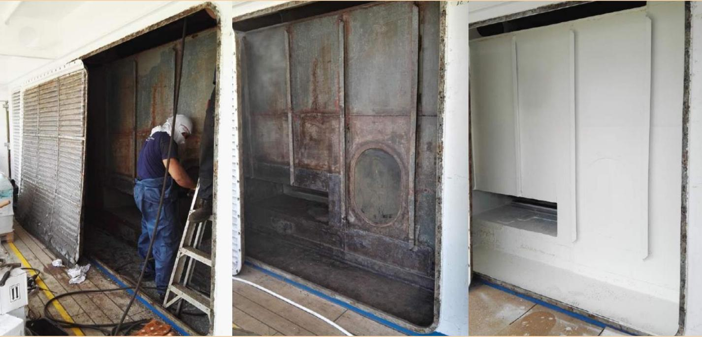
Our **turnkey service** for external **intakes** includes: chipping and cleaning the corrupted surfaces, **MAD Bond** applied to stop corrosion, **MAD Fiber** applied to restore damaged areas, painting the intakes with **MAD Armor**.
