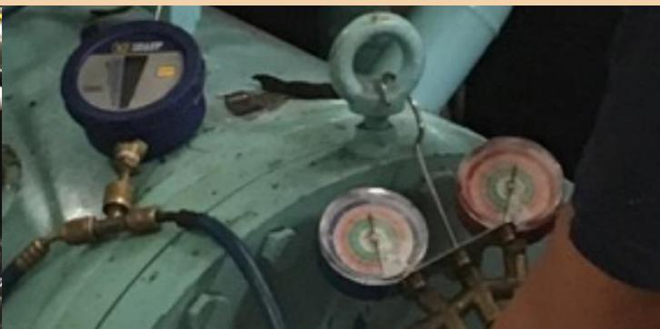
Nitrogen pressing of the circuit, just in case of leaks undetected neither by soapsuds nor by the leak detector device.
